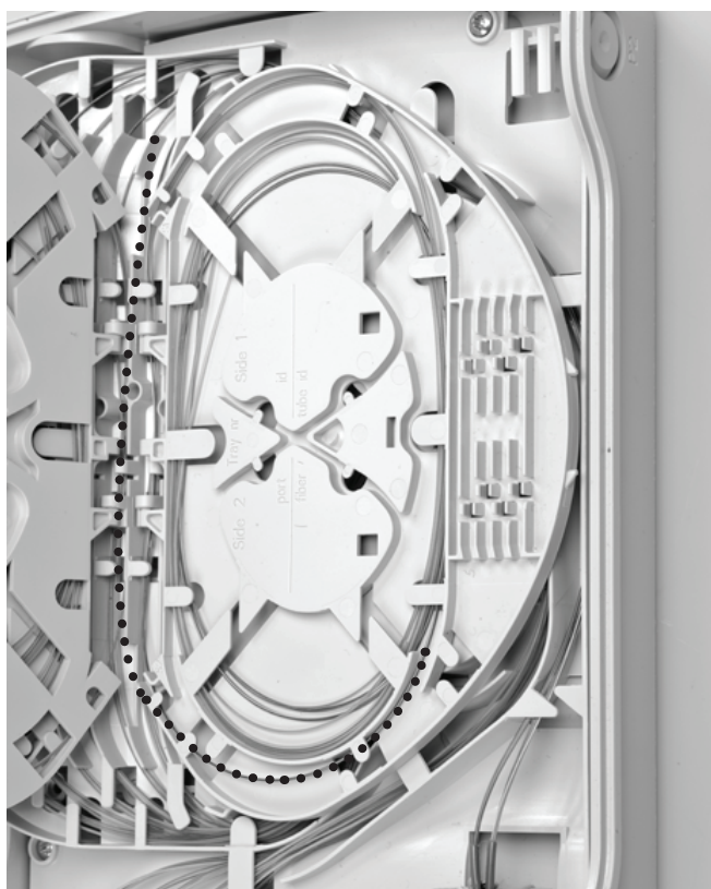
3.12 Route the fibers of the feeder cable towards the splicing trays.
