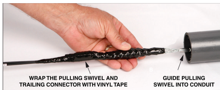
Figure 4. Vinyl Tape and Conduit
