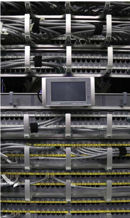
The NYU Shanghai project utilizes the SYSTIMAX imVision intelligent wiring management system across all three installations. Combined with patch panel monitoring hardware and system software, the imVision system provides a wide range of features and functionality to improve system management and lower maintenance costs.
