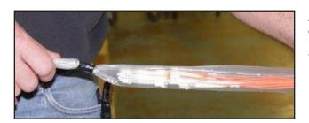
After you have pulled the fiber and power conductors into the OVP box remove electrical tape from the trunk cable and remove clear tube for access to all optical connectors.
