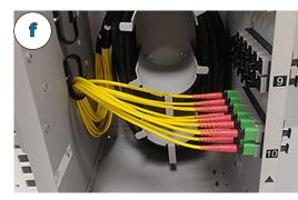
(f) Use retention clips to hold trunk subunits to left side of cabinet, ensuring that a drip loop of yellow connector tubes is formed toward rear of enclosure.
