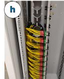
(g) Route next 6 subunits (labeled #5 - #7) to bottom middle set of radius limiters; wrap and connect.
