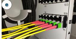
(e) Connect trunk subunits to corresponding connector numbers exactly per IDs on bulkhead. For example, connect longest subunits labeled 115-120 to adapter pack #10 in bottom half of enclosure.
